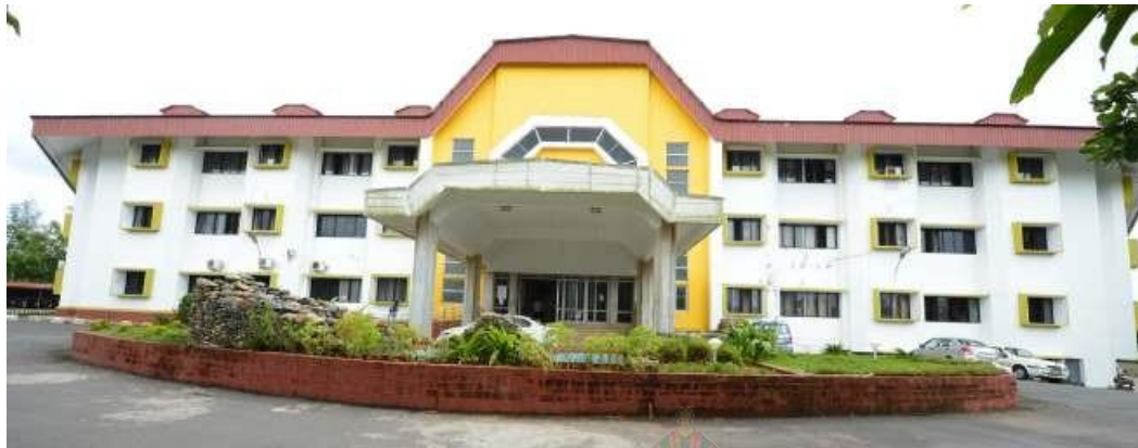
University Administrative Building
