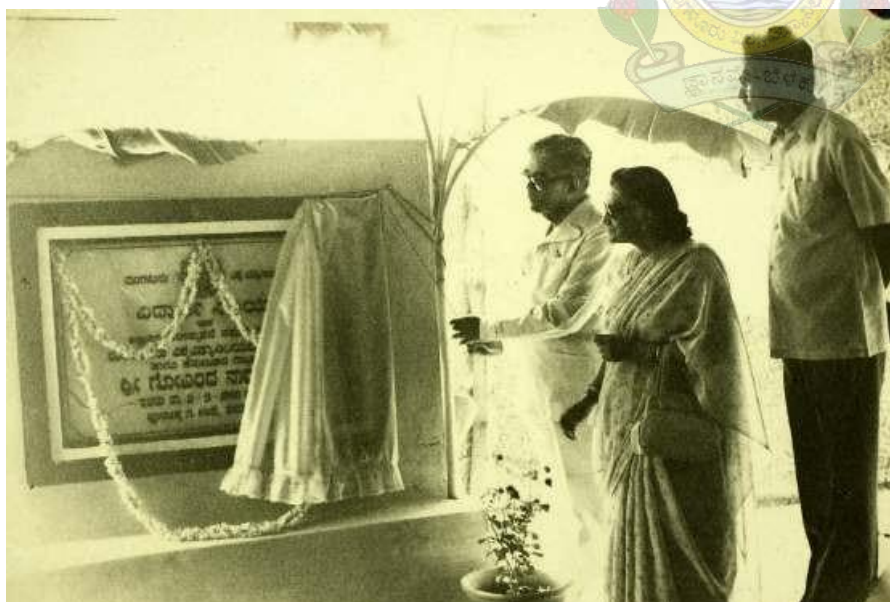
His Excellency Governor of Karnataka Sri Govindanarayana laying the foundation stone for Boys Hostels
